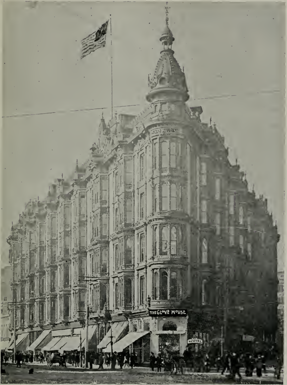
PHELAN BUILDING 806 Market Street
